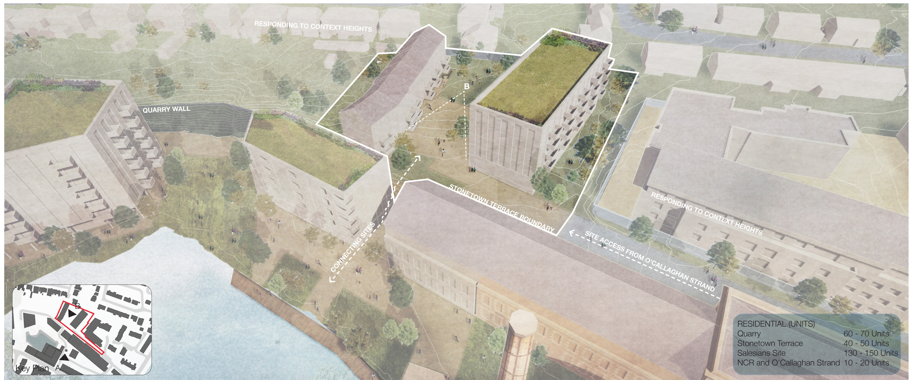
A - Aerial overlooking Stonetown Terrace
